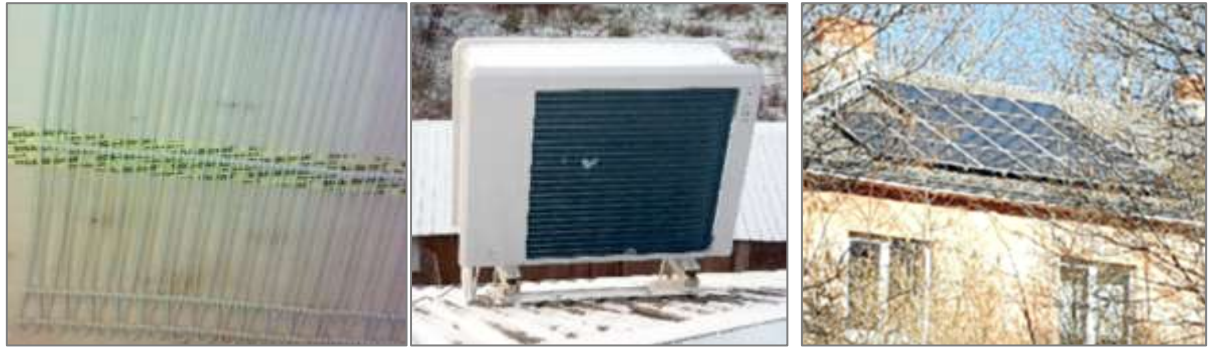
Figure 3. Components used in a studied apartment – capillary mats, heat pump and solar panels (see also Fig. 4).
