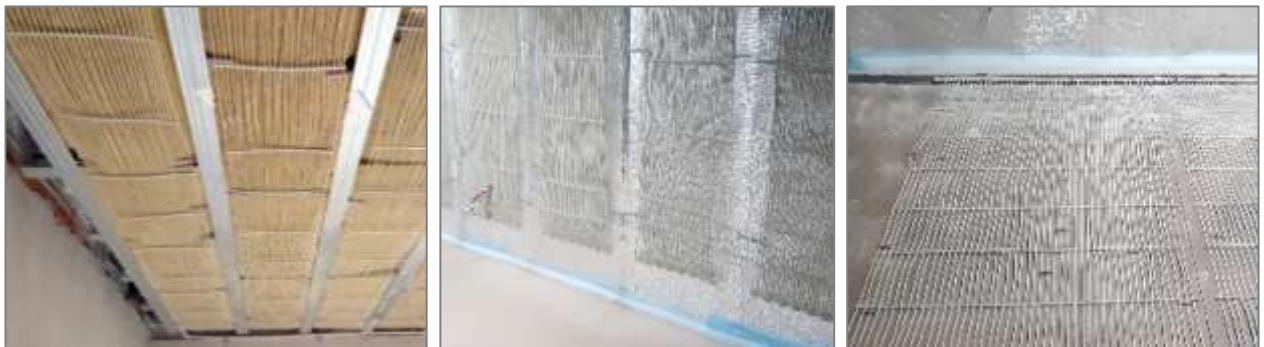
Figure 6. Capillary heat exchangers installed in ceiling, walls and floor.
